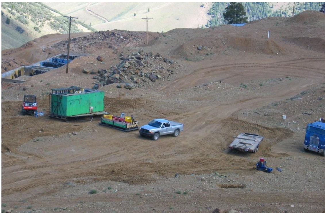
Figure 7 Drill Activity at Empire Mine Project
