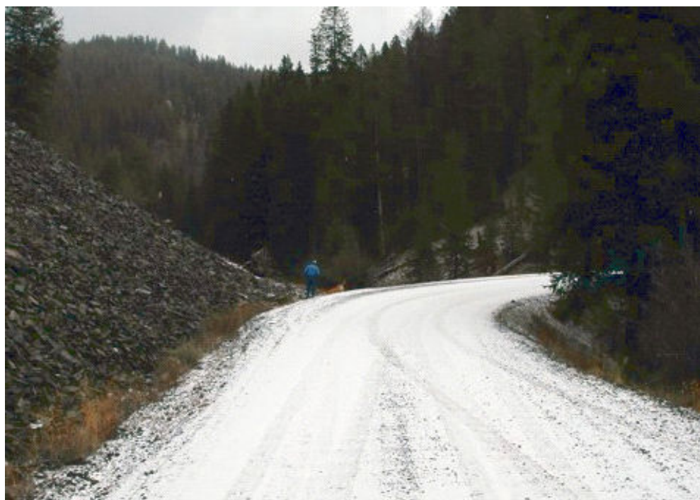
Figure 9 Well Maintained Access Road
